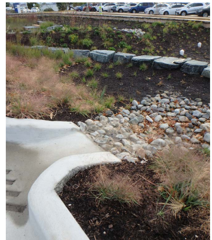
Recently installed bioswale in a parking lot.
