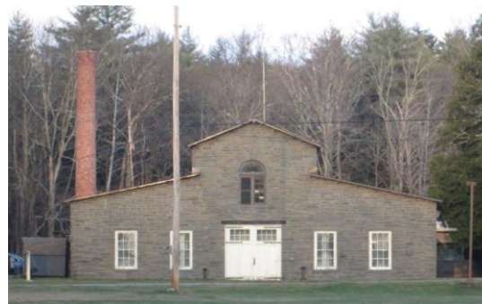
Edmund T. Cloonan Water Treatment Plant
