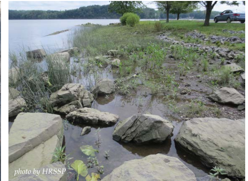
This shore zone is protected by lines of riprap and vegetation rather than an obtrusive wall.
