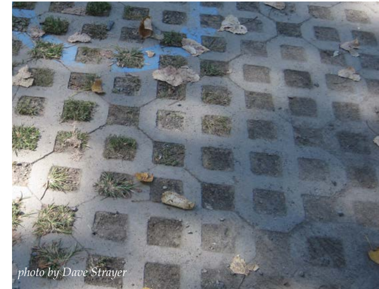
Permeable paving used in a parking lot.
